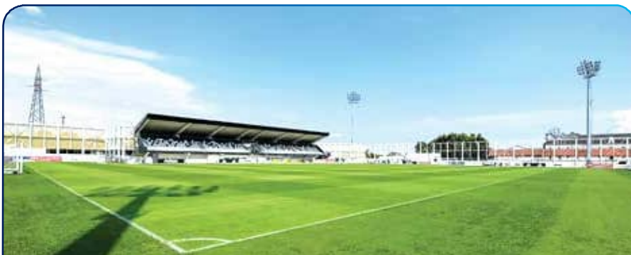
Figure 51. Example of floodlighting (International)
